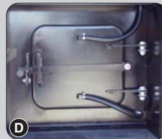
Awkward door location makes lighting a fire, loading wood, and cleaning out of ashes with a shovel (when the auger fails) a hassle.
