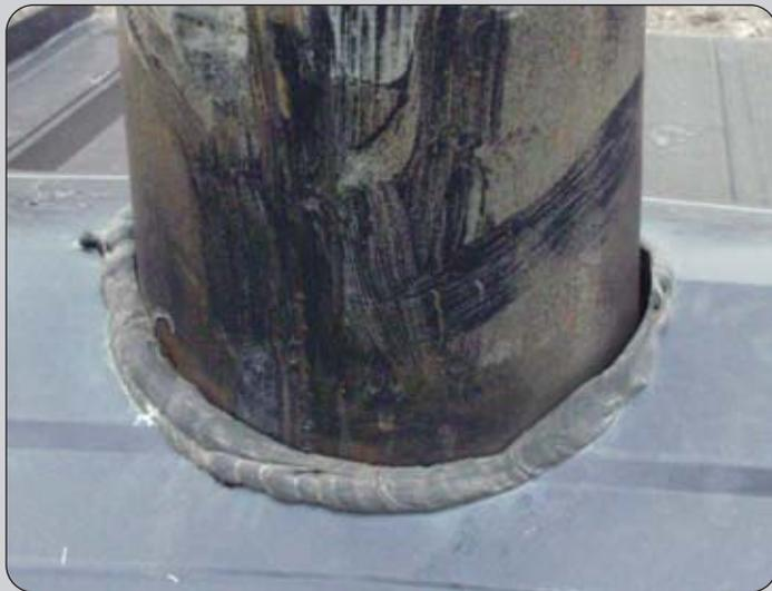
This illustration shows a chimney exiting out the top of a furnace through the tin roof. With this design, the high chimney temperature causes the caulking to loosen or burn off. This results in moisture penetrating the enclosure causing corrosion to the water jacket, chimney base, and a depletion of the fiberglass batt insulation's R-value.
